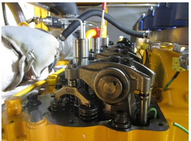
Service Motor BHKW
